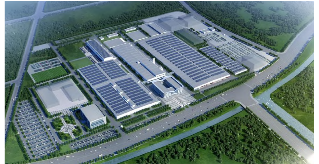
Zhaoqing Plant's Photovoltaic Carport and Roof Power Generation Project
